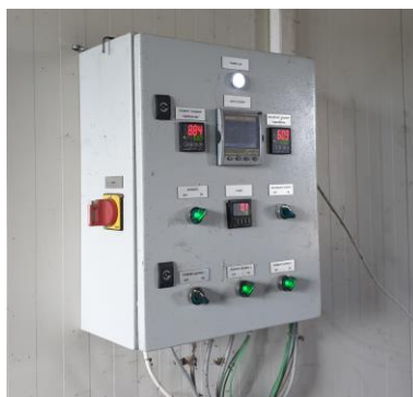
Fig. 8. Sampling point for biohazards on the crane control panel
