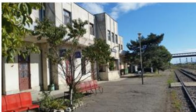
Fig. 3. Railway station Timisoara Sud.
