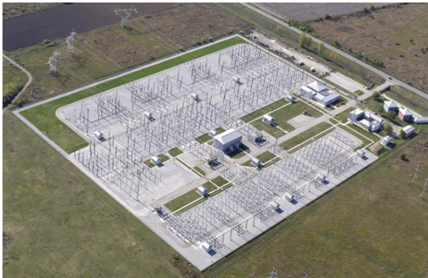
Fig. 3. Bird's-eye view of the TS 400/110 kV Ernestinovo, source [7]
