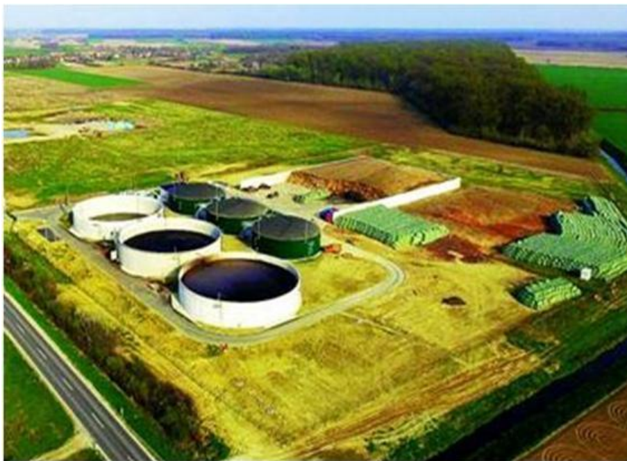
Fig. 4. Biogas power plants (2 MW) "Biointegra" Slatina, Croatia [8]
